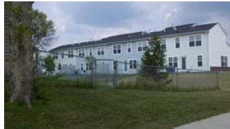
Needs weeded at fence line
