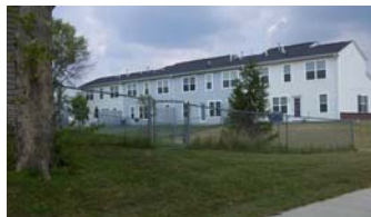
Needs weeded at fence line
